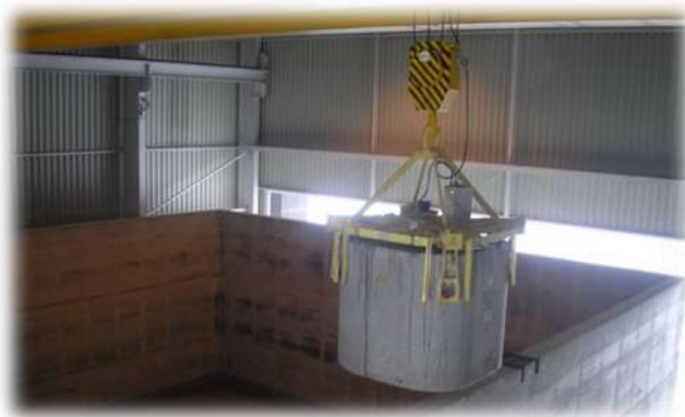
Figure 16. Loading of Radwaste Package into ENSDF Compartment
