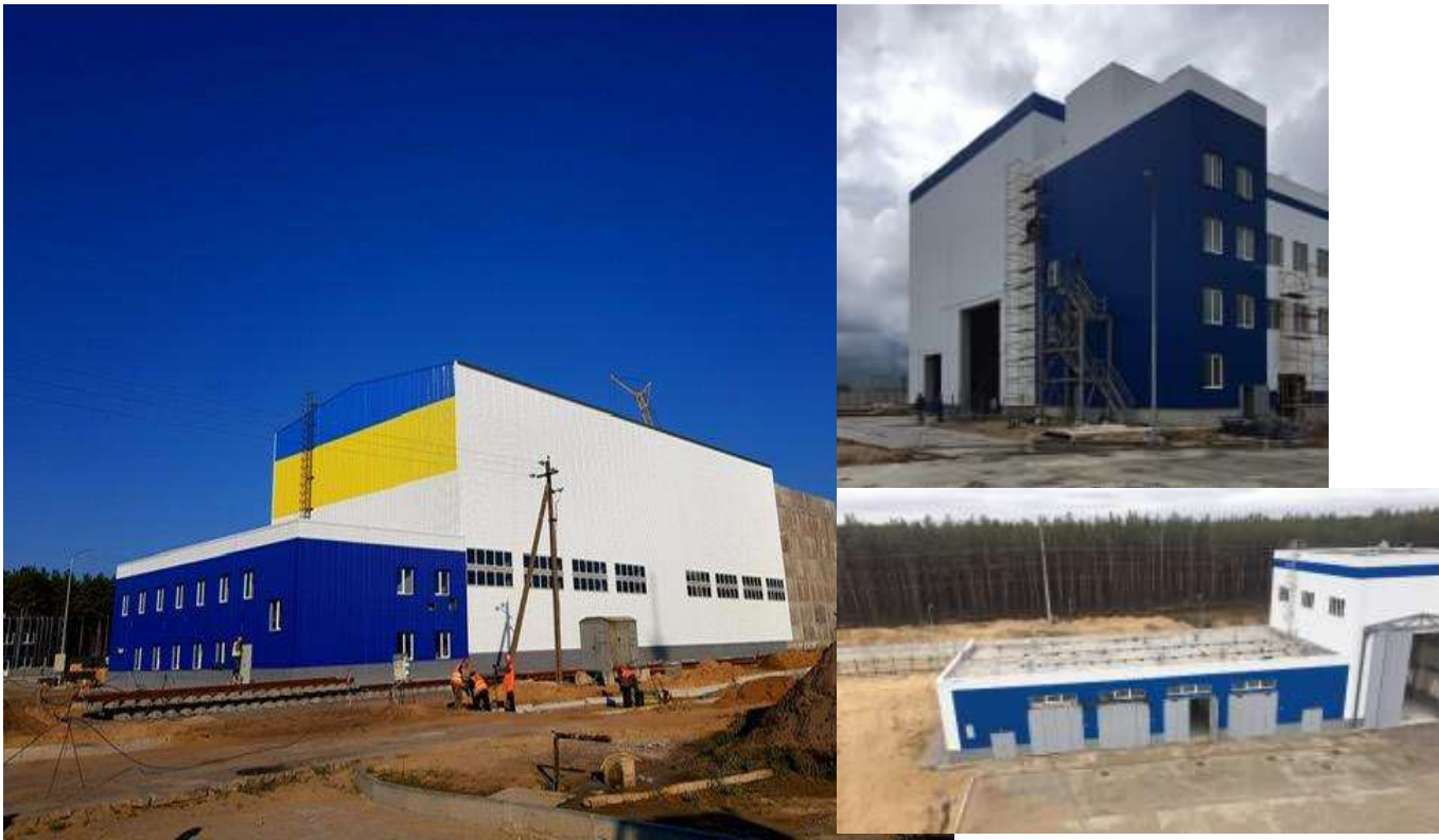
Figure 2. CSFSF Construction Site
