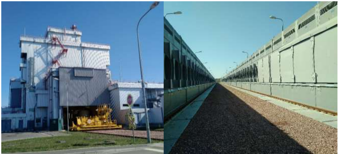
Spent Fuel Treatment Facility before Storage, ISF-2
