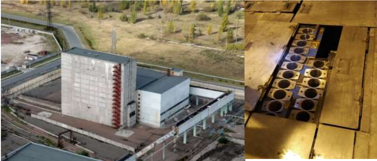
Figure 3. Wet Spent Fuel Storage Facility (ISF-1) of ChNPP
