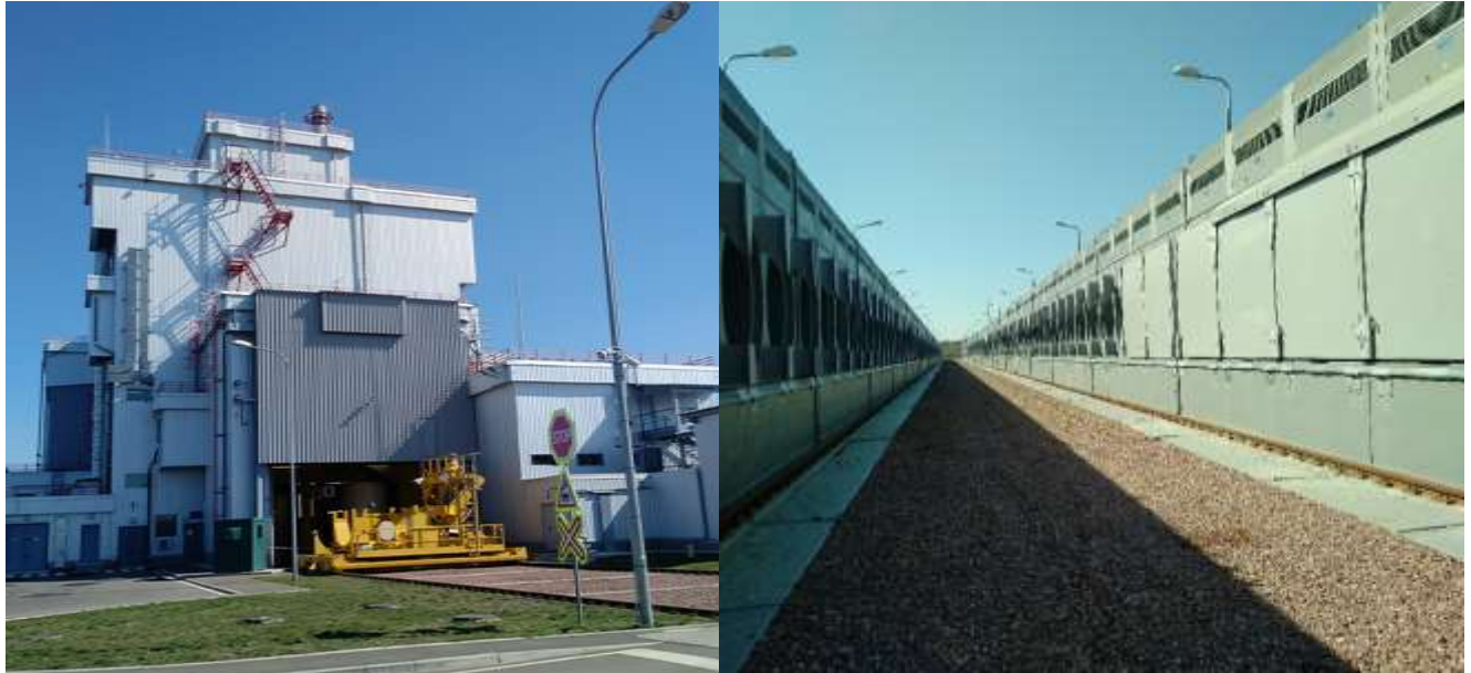
Spent Fuel Treatment Facility before Storage, ISF-2
