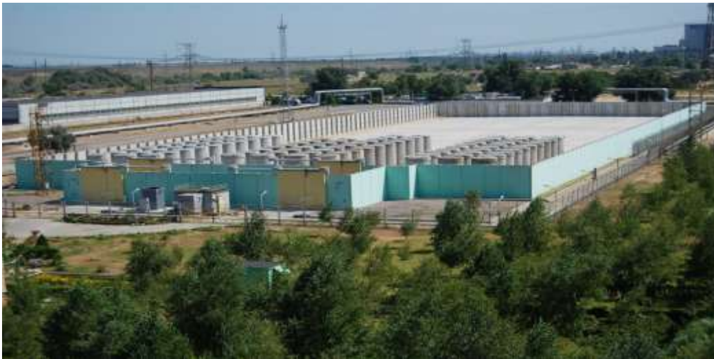
Figure 1. ZNPP Dry Spent Fuel Storage Facility (DSFSF)
