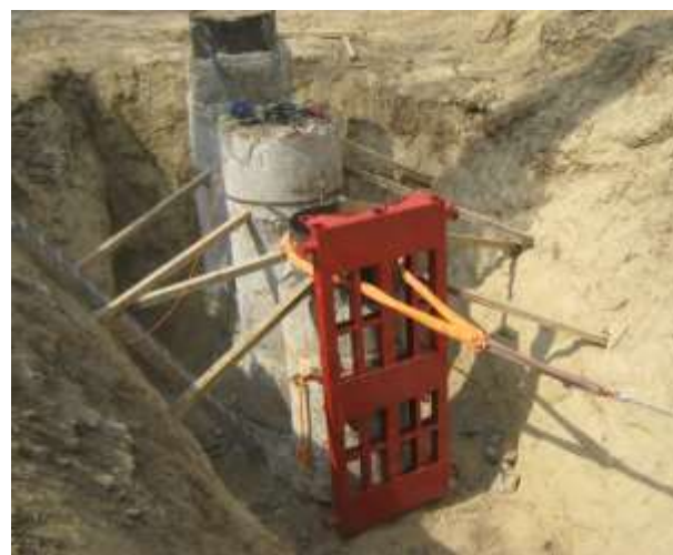
Figure 24. Radwaste Retrieval from Tsybuleve Facility
