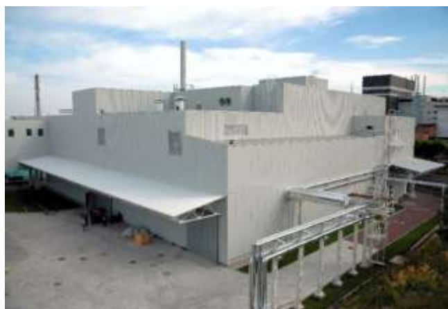
Figure 9. Solid Radioactive Waste Treatment Plant at ChNPP
