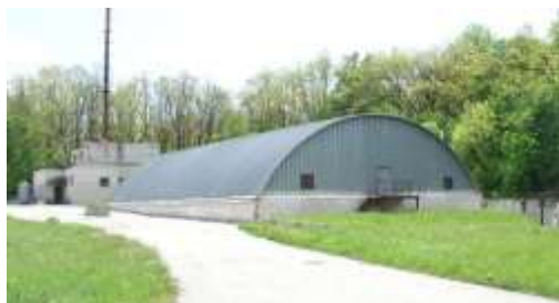
Figure 21. Container Storage of Radwaste in Hangar-Type Facilities
