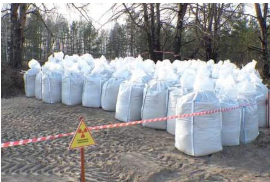
Figure 22. Preparation of Radwaste Retrieved from RWDS Pisky-1 for Transfer to Disposal
