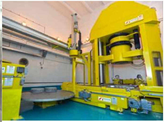
Figure 7. Solid Radwaste Supercompaction Facility, RNPP
