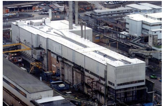
Figure 38: Magnox Swarf Storage Silo
