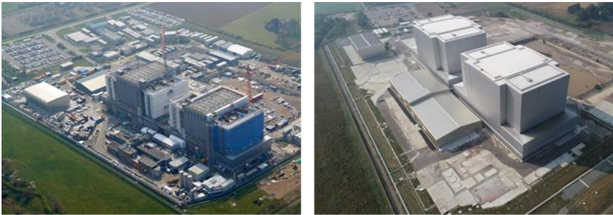
Figure 48: Bradwell during C&M preparations (left). Bradwell in C&M (right)
