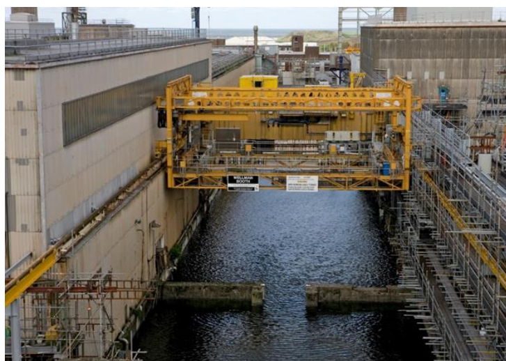
Figure 28: First Generation Magnox Storage Pond
