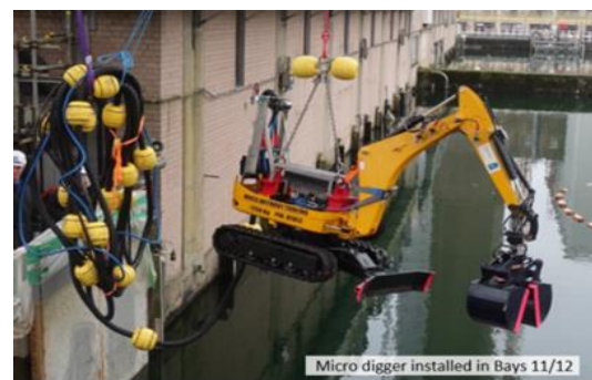
Figure 36: A micro-digger used to clear solid debris from PFSP bays 11 and 12.
