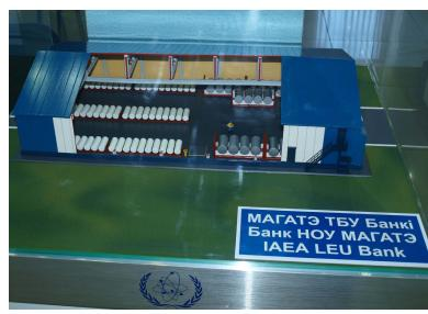
Model of the IAEA LEU Storage Facility being established in the Ulba Metallurgical Plant in Ust-Kamenogorsk, Kazakhstan.
