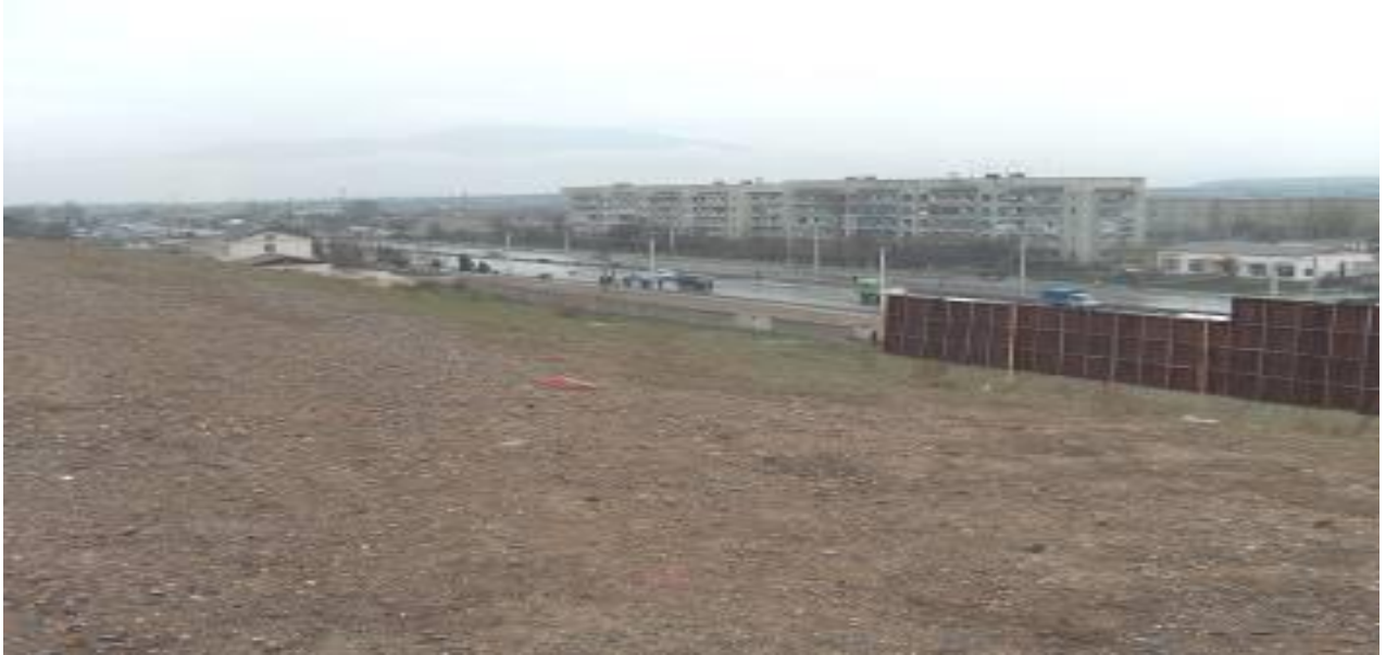
Gafurov tailings site: Note the proximity of dwellings, the cover appears intact with no obvious erosion features
