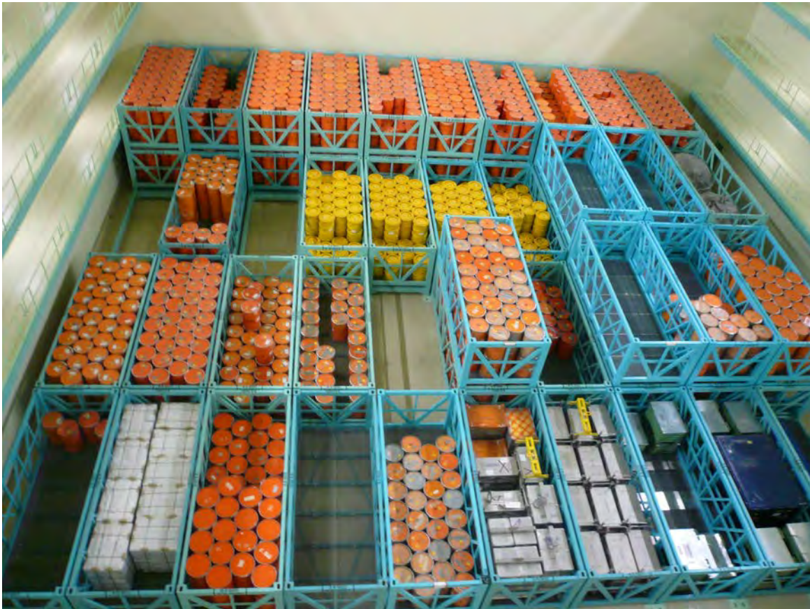
Figure 11: Storage hall for the storage of low level operational waste ZWIBEZ (Photo: ENSI)
