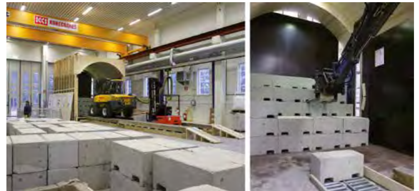
Figure A15 The Multi-purpose Test Facilities at Äspö. The photo shows the testing of a self-positioning robot for backfilling a deposition tunnel with bentonite blocks.
