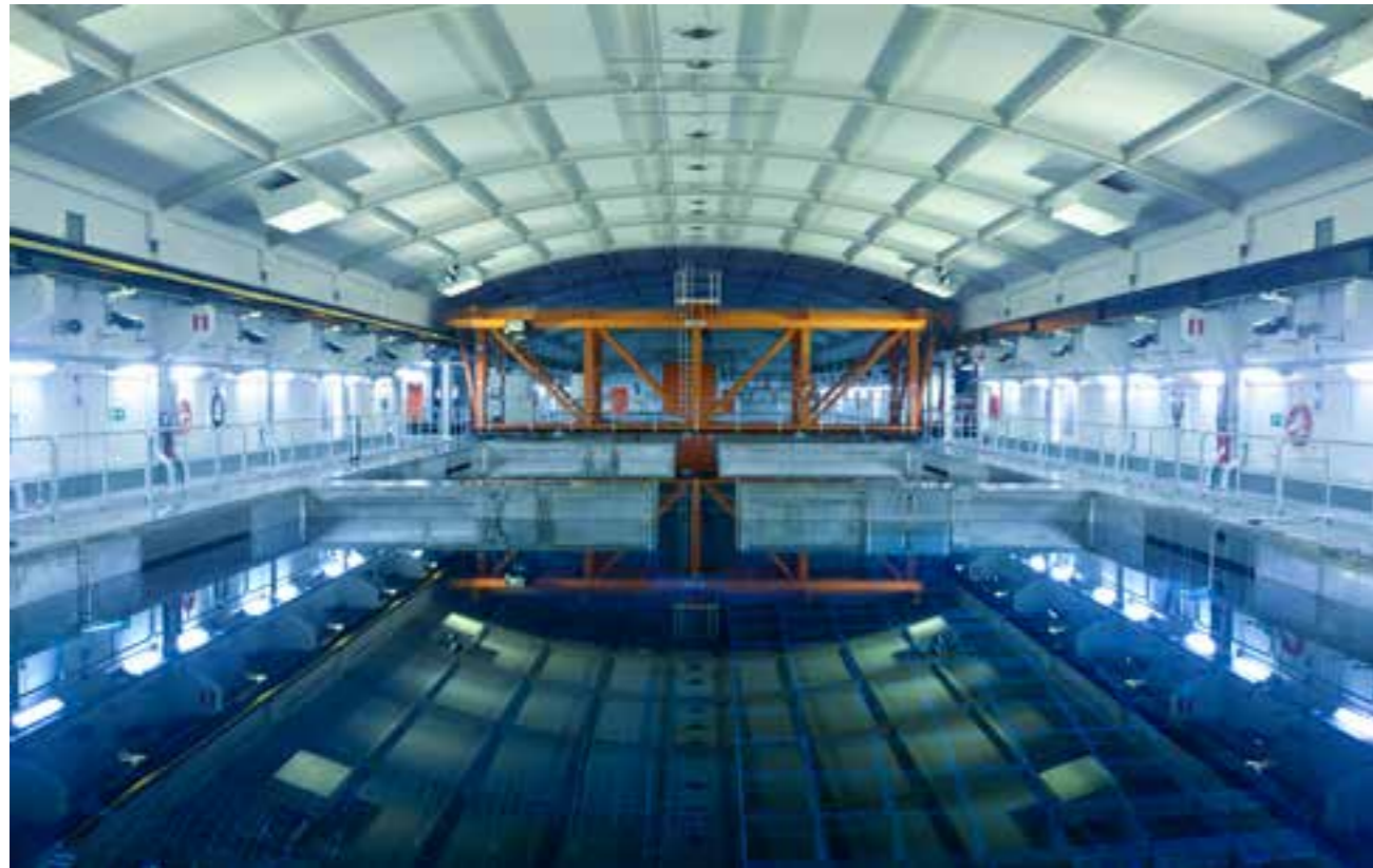
Figure A4 Storage pool in Clab. The top edge of the spent fuel is eight metres below the water surface.
