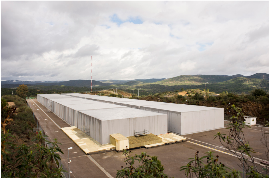
Image of the LILW disposal vaults at the El Cabril Disposal Facility.
