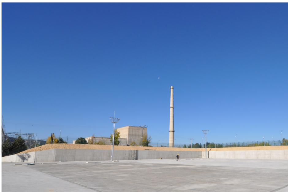
Overview of the Santa María de Garoña Nuclear Power Plant ITS.
