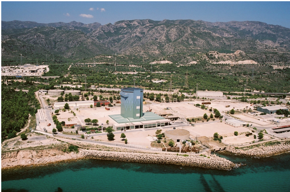
Image of the Vandellós I Nuclear Power Plant under decommissioning, currently in latent period.
