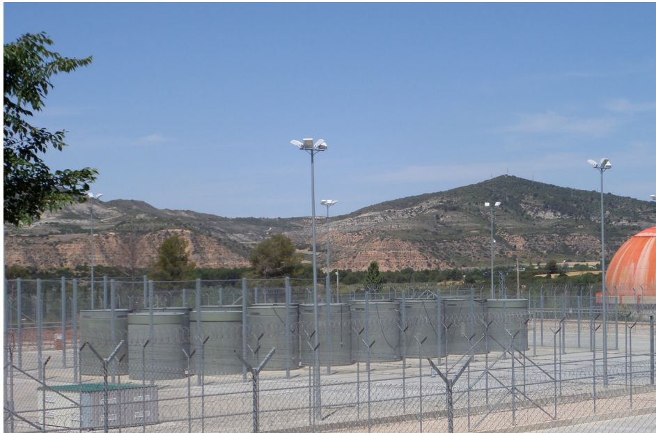
Overview of the José Cabrera Nuclear Power Plant ITS.
