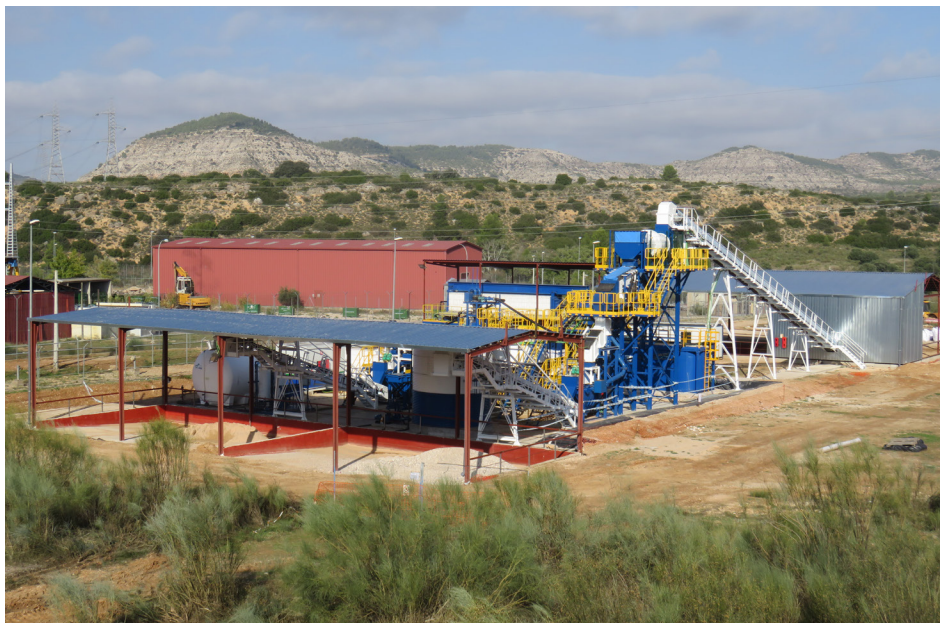
Image of the soil treatment plant at the José Cabrera Nuclear Power Plant.
