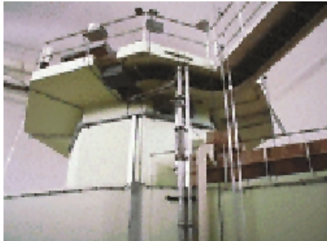
Figures 11 and 12: The reactor body and the reactor tank of the TRIGA Mark II research reactor.
