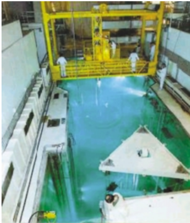
Figures 7 and 8: The Krško NPP fuel transfer channel and Westinghouse PWR fuel element.
