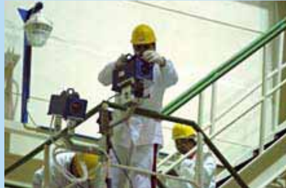
All in One Surveillance Unit or commonly called ALIS is a fully self-contained digital surveillance system. ALIS are normally mounted at high levels to give a clear activity view and provide a good recording of activity within the reactor hall.
