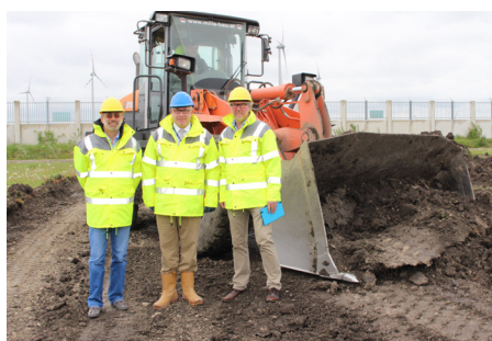
Start of FML excavation works in April 2017
