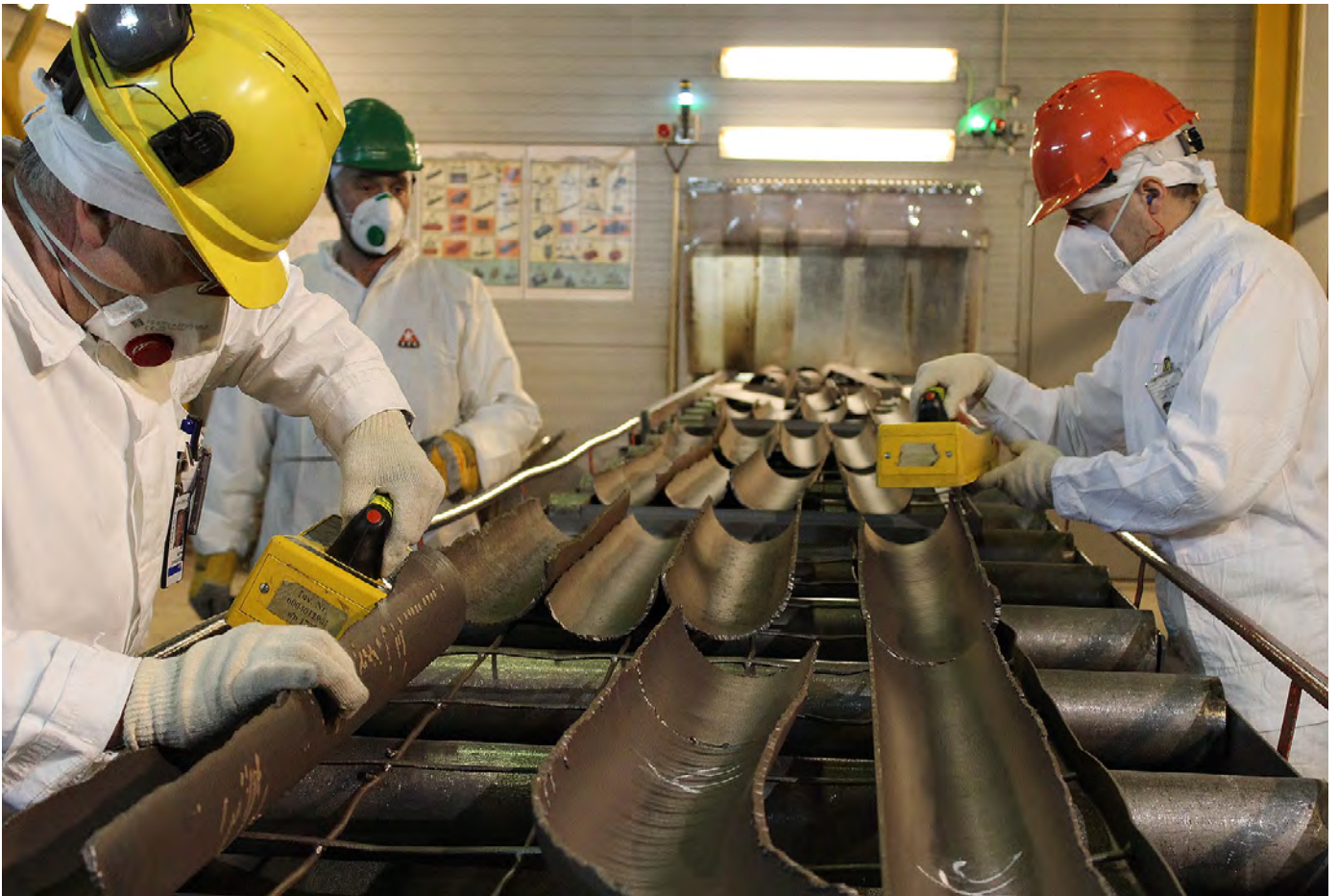
FIG. 2. Workers dismantling the turbine hall at Ignalina nuclear power plant measure scrap metal for traces of radiation (file photograph).
