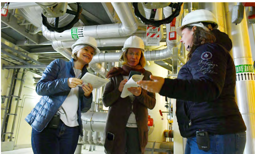
FIG. 2. Participants in the Hands-on Regulatory Inspector Training Workshop for Member States embarking on a nuclear power programme at the Zwentendorf nuclear power plant.
