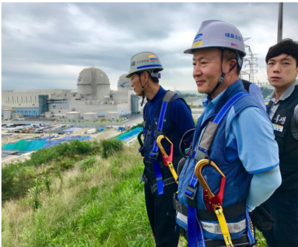
Experienced managers overlooking the construction of multi-unit Shin-Kori nuclear power plant.
