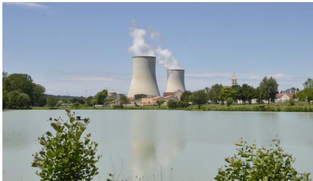
Civeaux nuclear power plant, France
