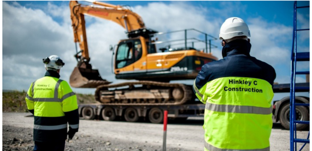
Workers at Hinkley Point C construction site
