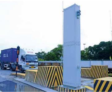
An RPM detects radiation in real time and does not interrupt normal export operations at the border. In addition, cameras simultaneously identify containers, capturing images of the truck and detailed information including plate and container number. The measurement and images are transmitted to the Central Alarm Station (CAS) for further review.
