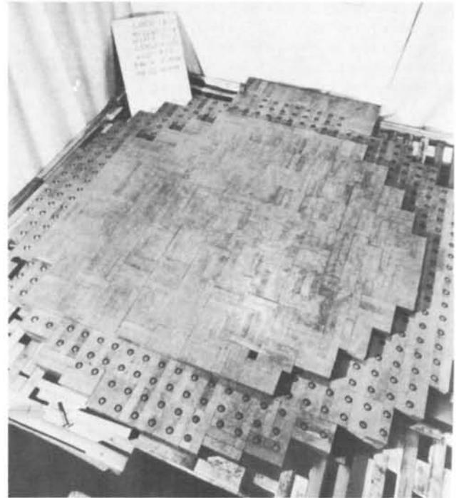
This is the only photograph of the world's first reactor taken during its construction at the University of Chicago. Taken in November 1942, the photograph shows the basic design of the pile, with alternate layers of graphite containing uranium metal and uranium oxide and spaced by layers of "dead" graphite (Photo Argonne National Laboratory)
