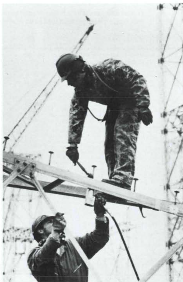
Workers on electric power lines. (Credit: EPRI)
