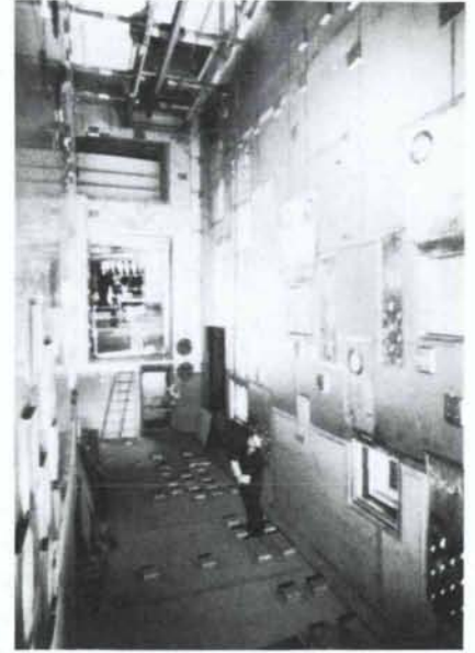
Inside the vitrification cell of the R7 facility being built at the Cogéma reprocessing plant in La Hague.
