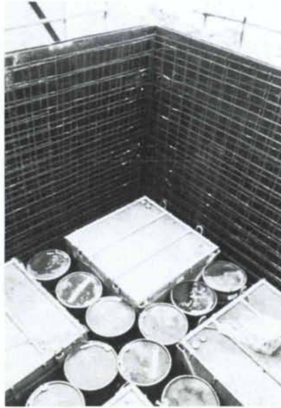
The bottom layer of a monolith at the La Manche disposal site: re-inforced walls and room for concrete grout.
