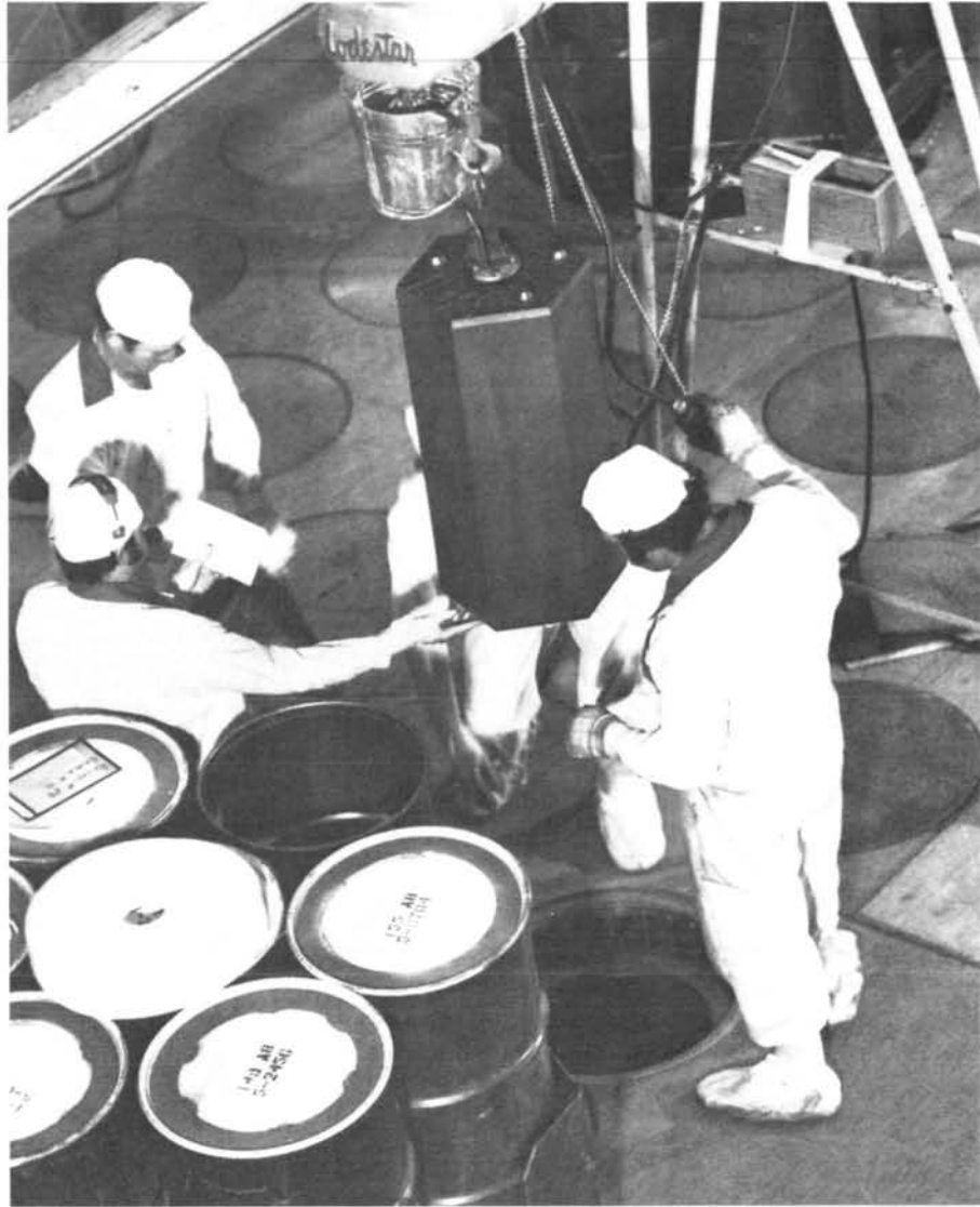
One of the 1482 graphite fuel blocks being lowered into the core of the 330-MWe Fort St. Vrain nuclear plant in Colorado, USA, the first commercial-size reactor using the advanced HTGR system. Since power generation began in 1976, the plant has generated more than 4 terawatt-hours of electricity. (Photo courtesy of GA Technologies Inc.).
