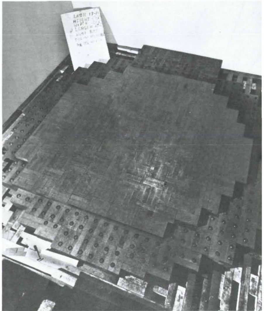
The nineteenth layer of graphite photographed during the construction of the Fermi Pile. Slugs of uranium oxide may be seen in layer 18 which is partly uncovered. (Photo: Argonne National Laboratory)
