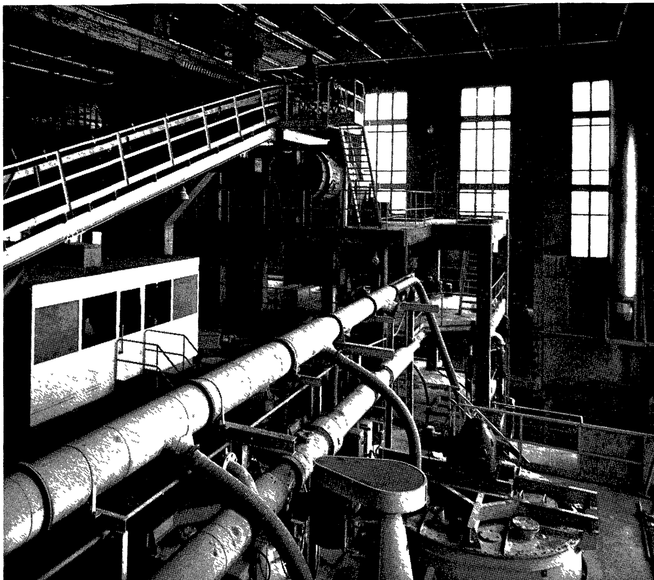
The interior of the ore-processing plant of l'Ecarpière in the Vendée region of France.
