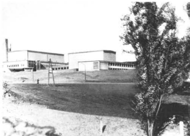
The reactor building at Vinca (Photo: Yugoslav Nuclear Energy Commission)
