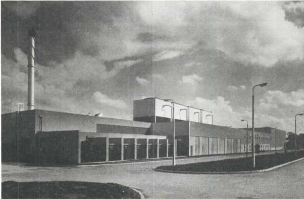
URENCO's production plant at Capenhurst, England. The plant uses the gas centrifuge process for the enrichment of uranium.
