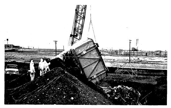
Rubbish which has low level radioactive contamination is loaded into a box, and dumped into a burial pit, at the Atomic Energy Commission's Hanford Works. It is being hosed to prevent possible spread of contamination by an errant breeze... Battelle-Northwest
