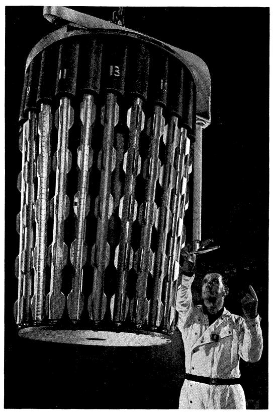
Herringbone type fuel elements being loaded into a fuel basket on the charge floor at Calder Hall.
