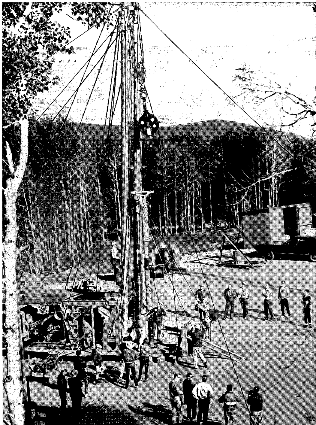
Before ... The 40-kiloton nuclear device used in Project Rulison is lowered into the emplacement hole. Photo: Los Alamos Scientific Laboratory
