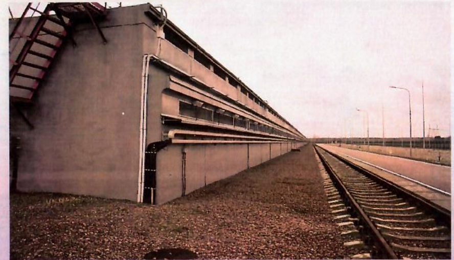
Concrete storage modules for spent fuel of the ISF-2
