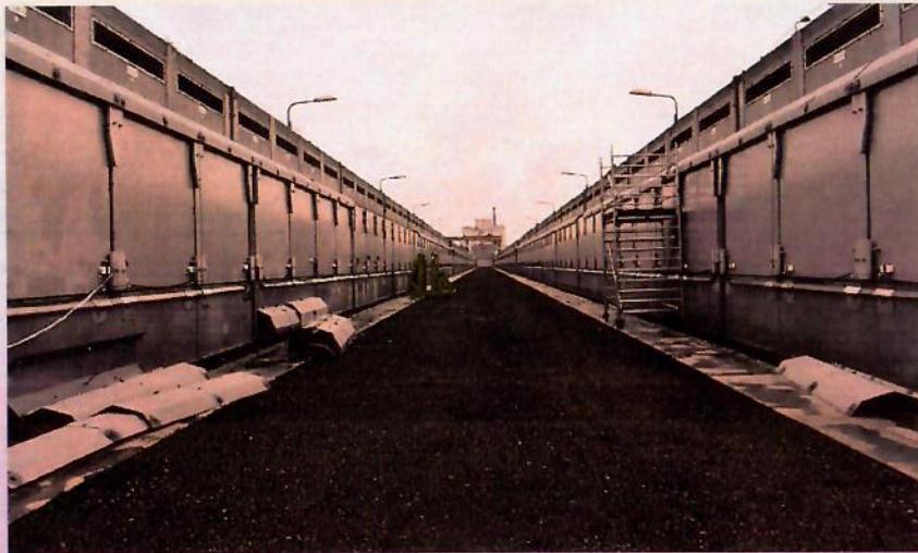
Concrete storage modules for spent fuel of the ISF-2
