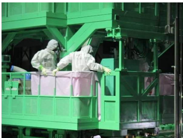
The NRA Safety Inspectors watch TEPCO's spent fuel removal operation on the fuel handling machine.
