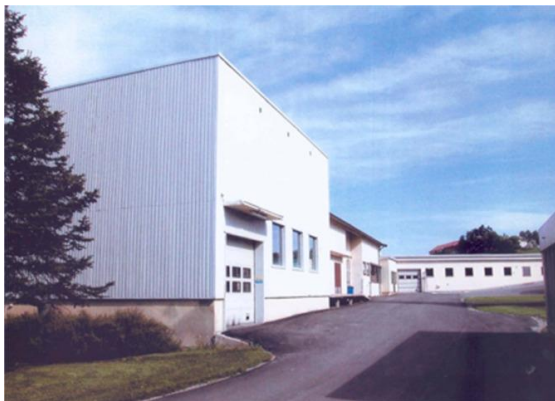
4-5 Radioactive waste facility, Kjeller site
