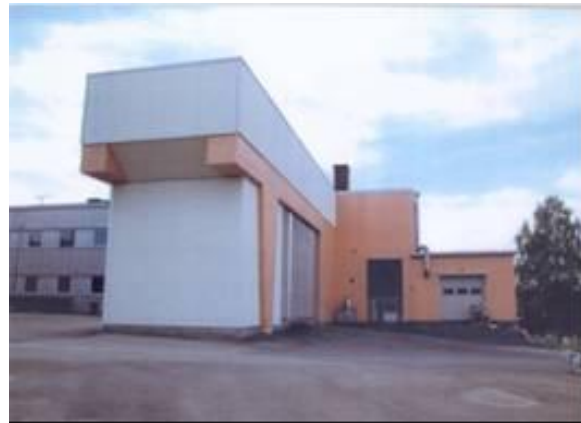
4-3 Spent fuel storage facility. Kjeller site
