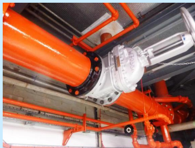
Figure 23 – Completed remediation on gas circulator fire pipework
