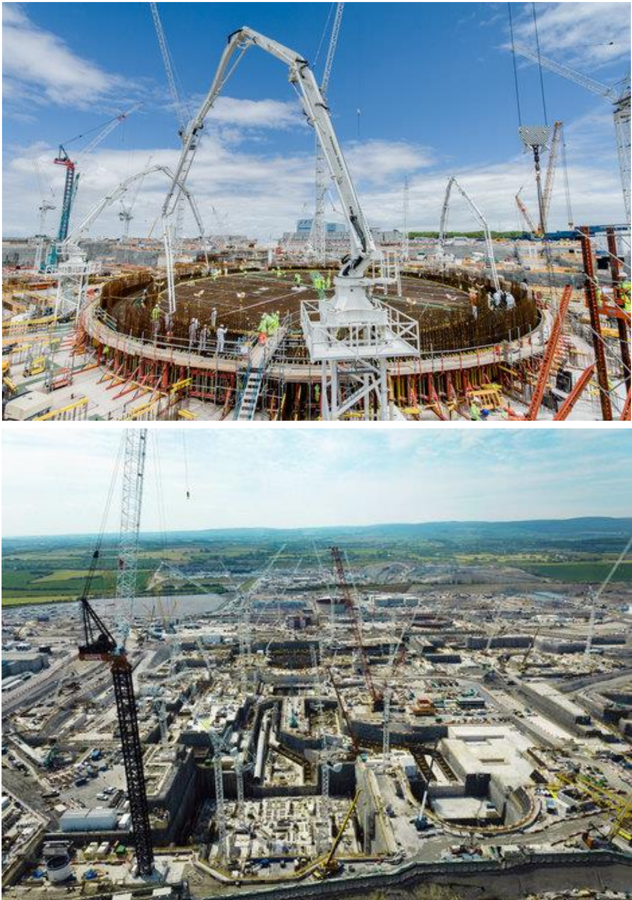
Figure 1 and 2 – Construction at Hinkley Point C
