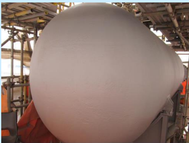
Figure 21 - CO 2 HP tank 21 during remediation
