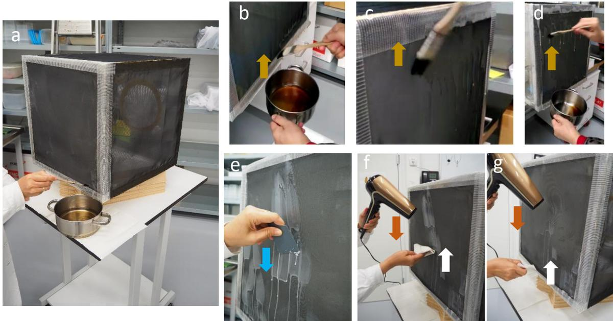
*Figure 3. Creating the wax panel. (a) Applying the wax; (b) (c) (d) Processing the bottom, the top and the centre of the cage panel; (e) Removing excess wax with a sharp tool; (f) (g) Equalizing the panel surface with a hair dryer. The arrows symbolize the direction of the different movements.*
