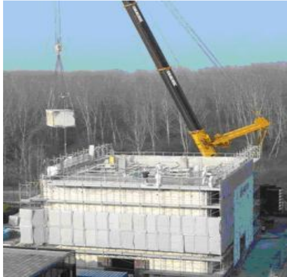
Figure 16: Caorso NPP - Off-gas building dismantling
