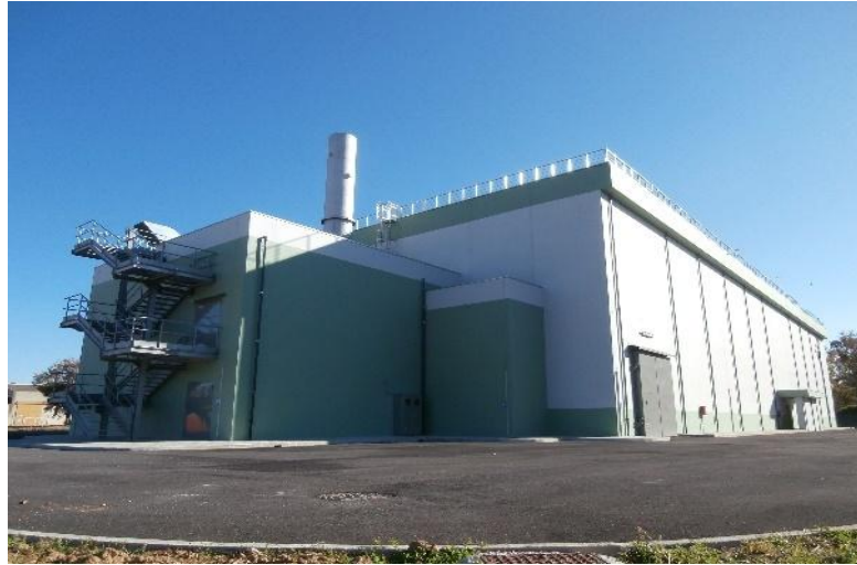
Figure 7: Latina NPP – New storage building
