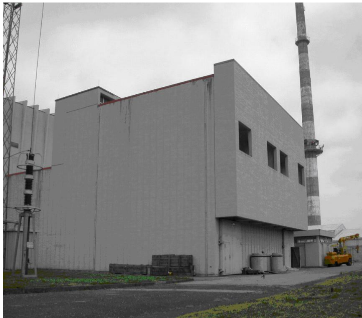
Figure 20: Storage facility “ex Diesel”
