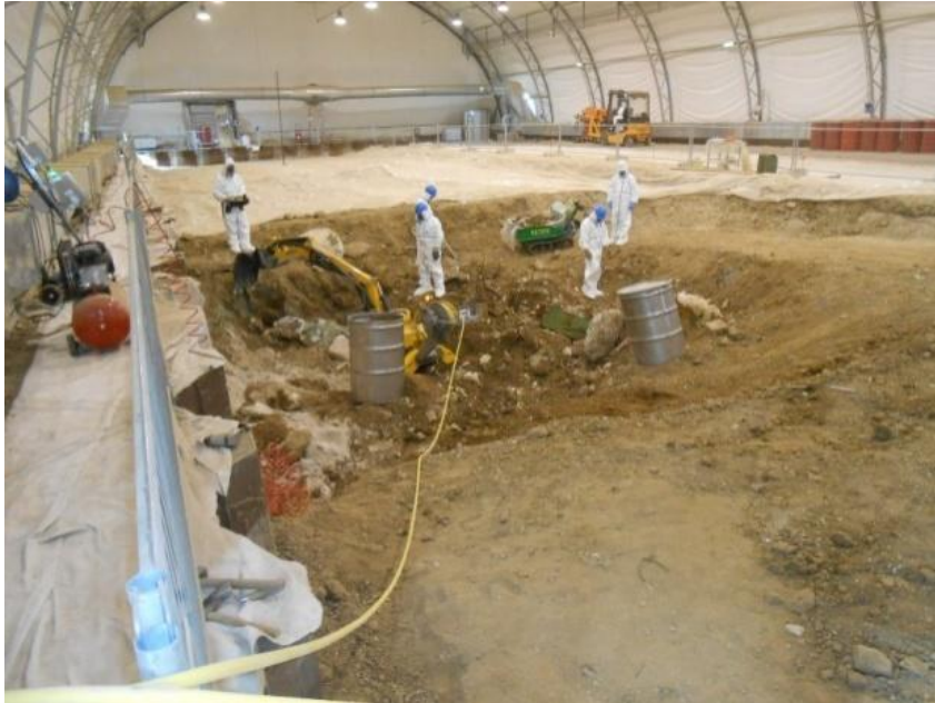
Figure 24: Trenches remediation activities
