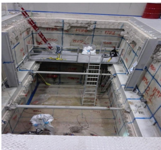
Fig. 44 Waste A&B – activity of radiological survey
