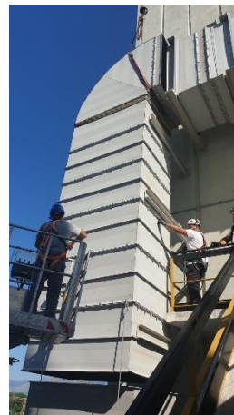
Figure 25: revamping of the ventilation system
