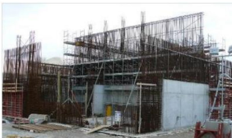
Figure 33: DMC3 and DTC3 construction
