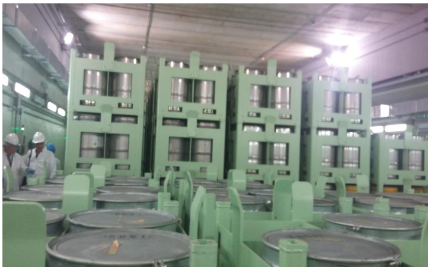
Figure 6: Garigliano NPP – D1 storage facility
