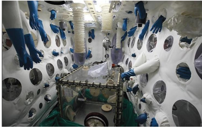
Fig. 45 Glove box dismantling at Plutonium plant
