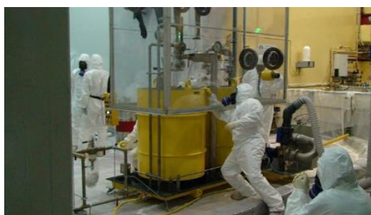
Figure 35: Cleaning of the bottom pool
