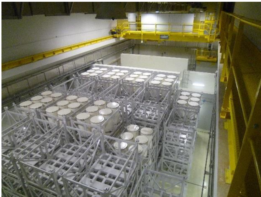
Figure 8: EUREX D2 storage facility
