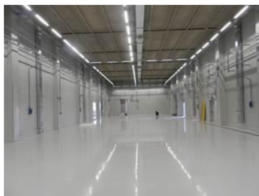
Figure 42: Refurbishing activities of building B106
