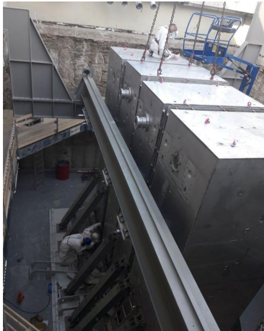
Figure 9: ITREC concrete block removal
