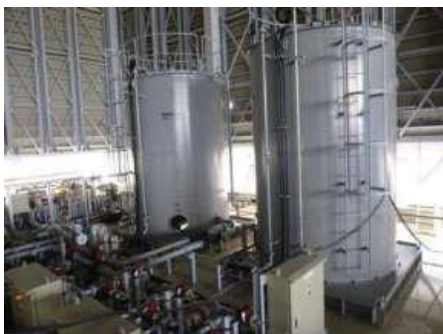
Figure 3: Installation status of additional multi-nuclide removal equipment
