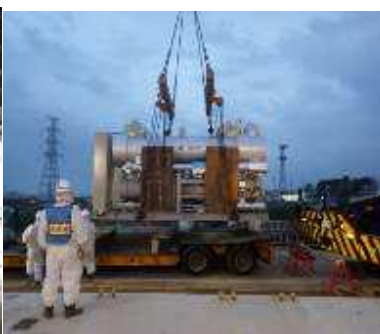
Figure 3: Installation status of additional multi-nuclide removal equipment
