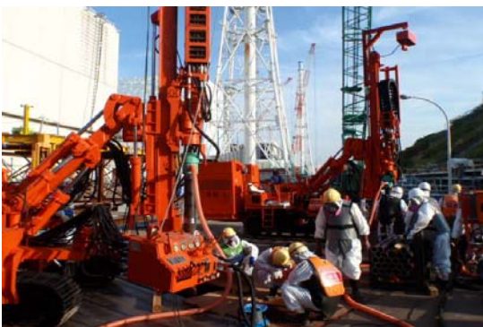
Figure 3: Installation of frozen pipes of land-side impermeable walls with frozen soil
