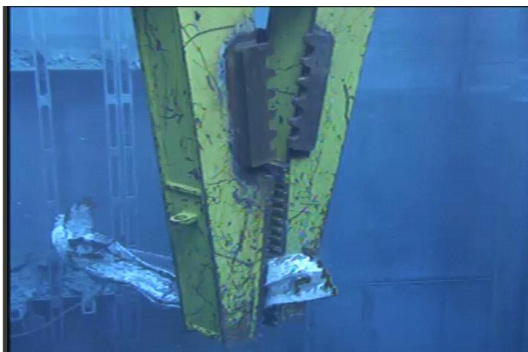
Figure 1: Rubble removal from SFP
