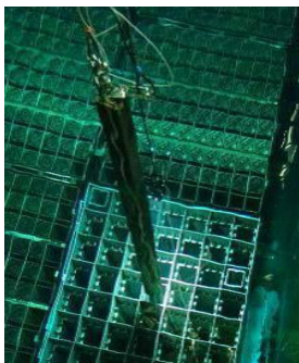
Figure 2: Spent fuel storage in common pool
