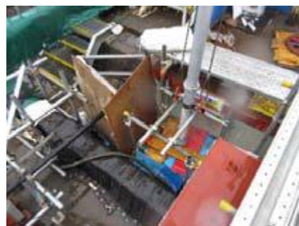
Figure 3: Hole for filling Unit 2 seawater-pipe trench tunnel sections
