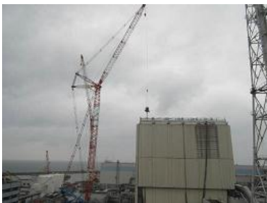
Figure 1: Opening of roof panel holes and spraying of anti-scattering agents
