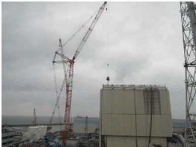
Figure 1: Opening of roof panel holes and spraying of anti-scattering agents
