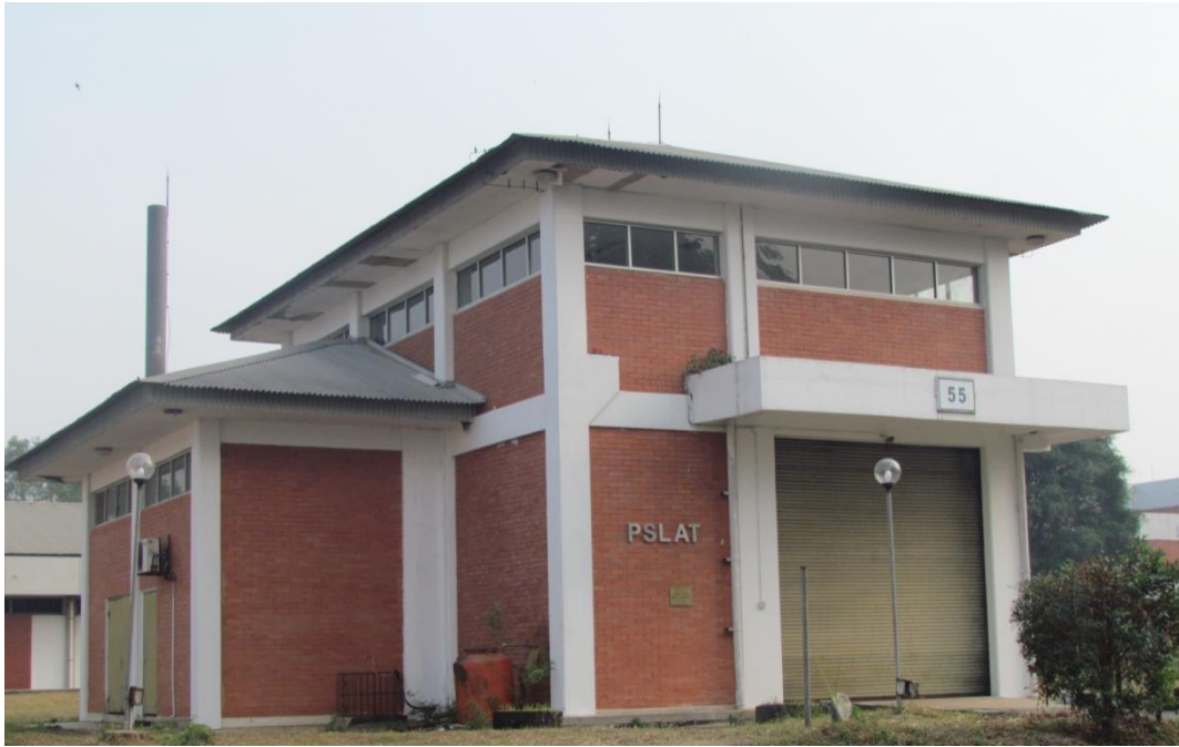
Figure 9. High Level Radiation Waste Building
