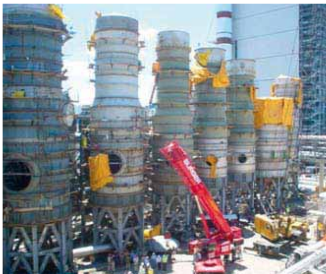
Cellulose plant under construction. Photo: Chilean Nuclear Energy Commission
