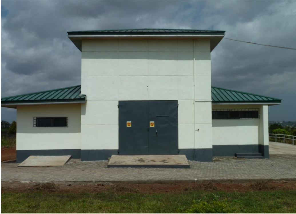
Figure 1a: Front view of the Centralised Radioactive Waste Processing Unit
