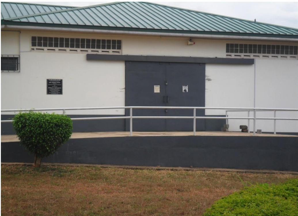
Figure 1b: Front view of the Centralised Radioactive Waste Storage Unit
