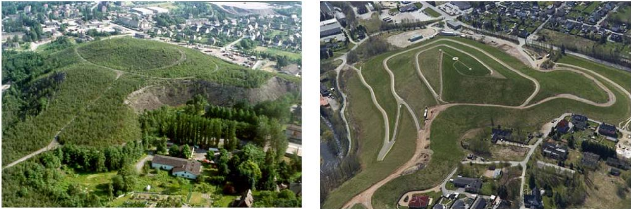
Fig. 1: Remediation of mine dump #66/207 (Schlema site, Edelhofweg area) before and after remediation
