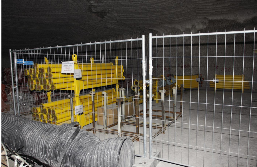
Figure F-7: Underground material storage at the 490-m level for an emergency in the Asse II mine (Copyright: BfS)
