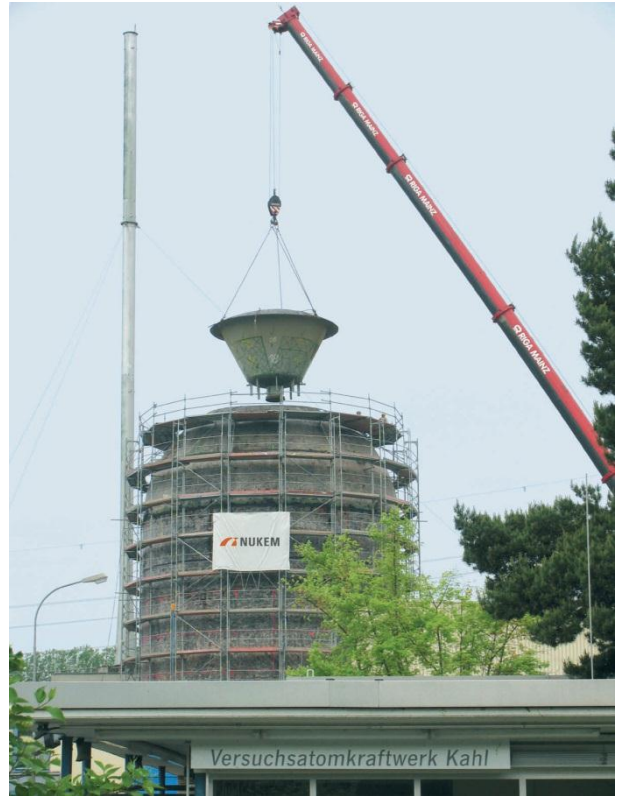
Figure D-21: The successive dismantling of the reactor building of the Kahl experimental nuclear power plant to the green-field (Copyright: NUKEM, BMU, RWE Power)
