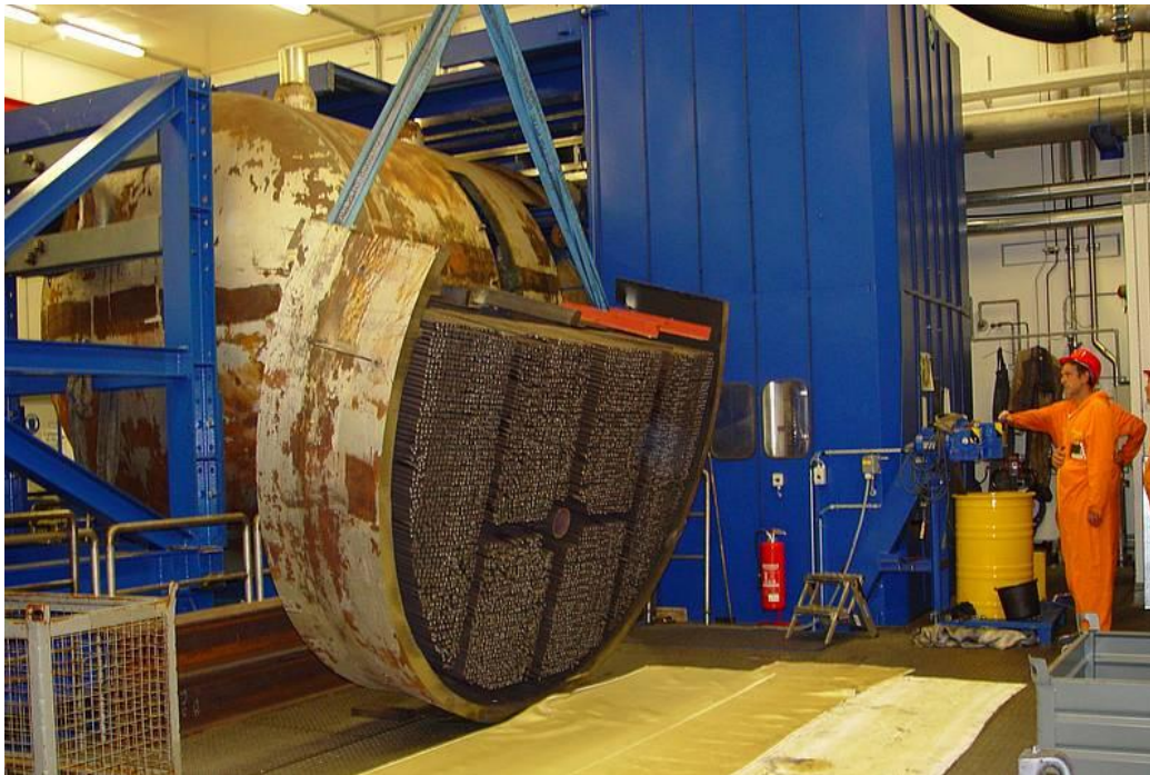
Figure D-20: Segmentation of a steam generator by sawing procedures in ZLN (Copyright: EWN)
