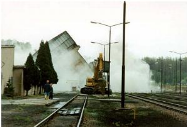
Fig. 6: Blasting of the Rottwerndorf ore loading facility (Königstein site) and the remediated plant areas
