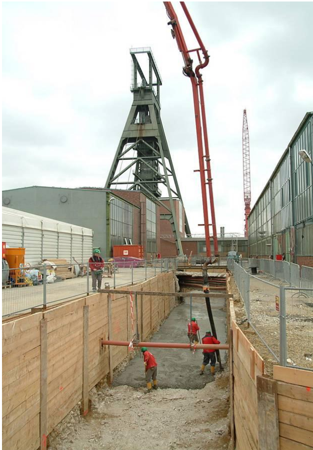
Figure D-15: Konrad repository in Salzgitter (left: underground media duct, right: basement of the building of the hoisting machine) (Copyright: BfS)
