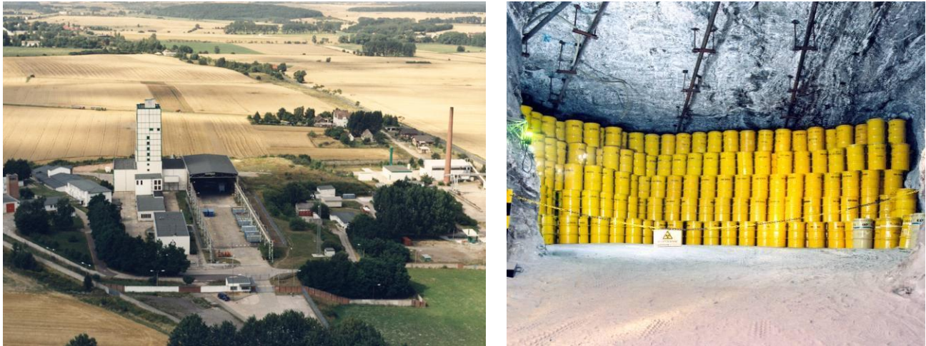
Figure D-14: Repository for radioactive waste Morsleben (ERAM) (left: aerial photograph, right: emplacement chamber with stacked drums low-level waste) (Copyright: BfS)
