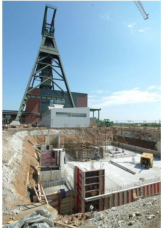
Figure D-15: Konrad repository in Salzgitter (left: underground media duct, right: basement of the building of the hoisting machine) (Copyright: BfS)
