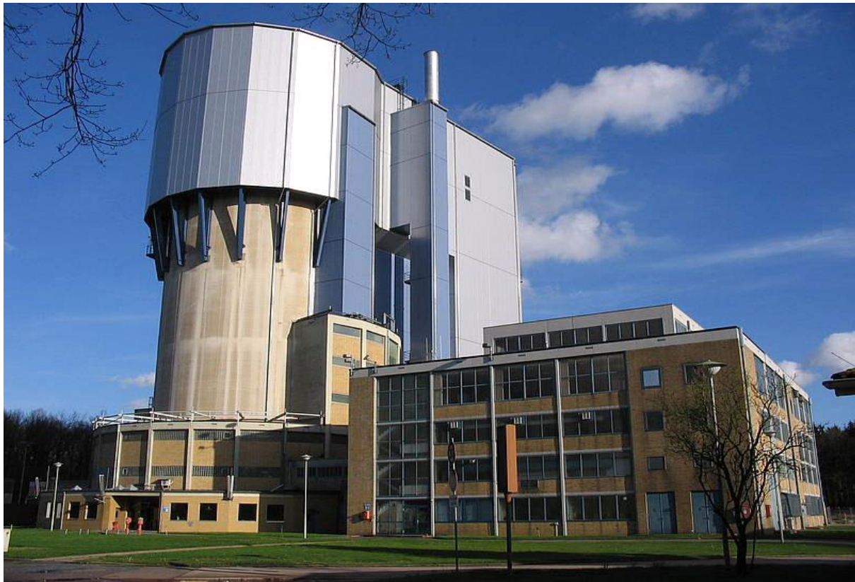
Figure D-22: Annex of the transfer building to the reactor building AVR (Copyright: EWN)
