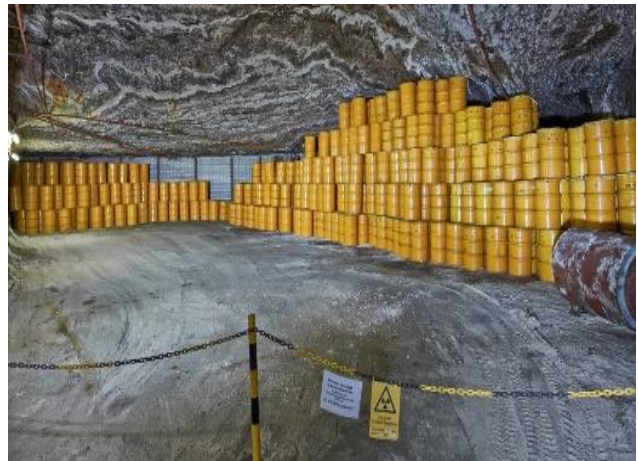
Figure D-8: Morsleben repository for radioactive waste (ERAM) (left: aerial view, right: emplacement chamber with stacked low-level waste drums) (Copyright: BGE)
