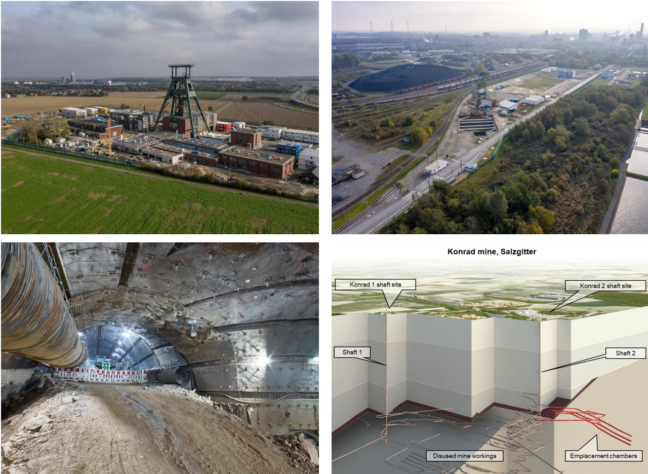
Figure D-9: Konrad repository construction site in Salzgitter (top left: Konrad 1 shaft site; top right: Konrad 2 shaft site; bottom left: Konrad Shaft 2, view into the inset on the second level; bottom right: graphic representation of the entire site (Copy-right: BGE))
