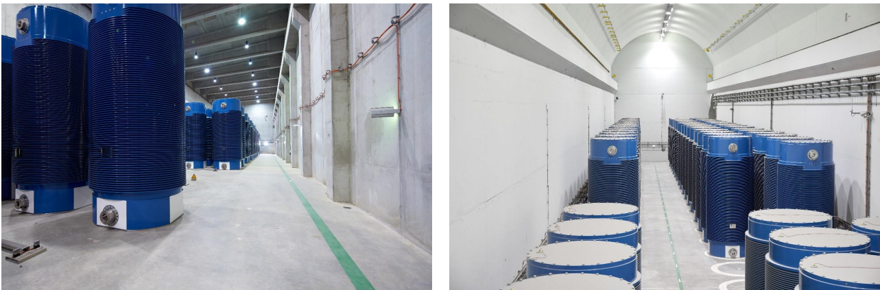
Figure D-1: View into the decentralised spent fuel storage facilities at the Gundremmingen (left) and Neckarwestheim (right) sites (Copyright: BGZ)
