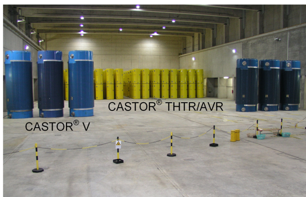
Figure D-5: Ahaus spent fuel storage facility (left: CASTOR® V and CASTOR® THTR/AVR, right: CASTOR® MTR 2 between CASTOR® THTR/AVR) (Copyright: BGZ)
