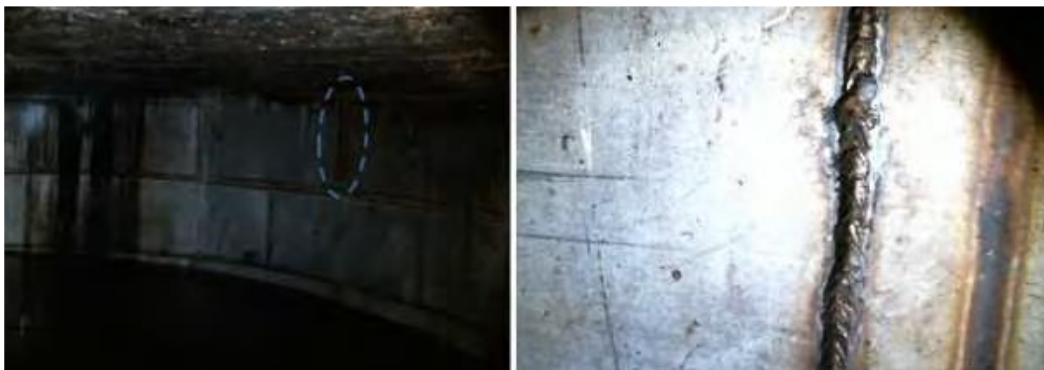
Fig.30 Inside view of the first tank
