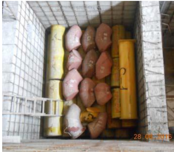
Fig.15 Decommissioning waste at TTR building vault
