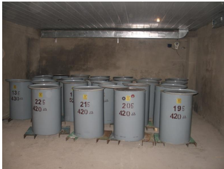
Fig.7 Drums with concreted waste
