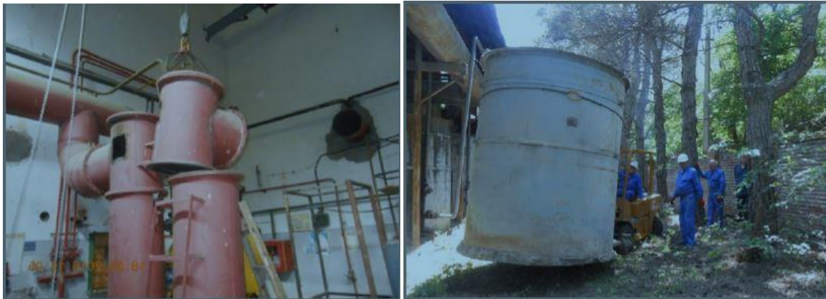
Fig.9 Dismantling of installations in cryogenic station
