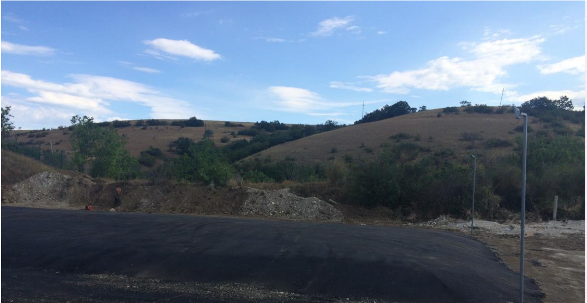
Fig.32 New cover of solid waste vaults
