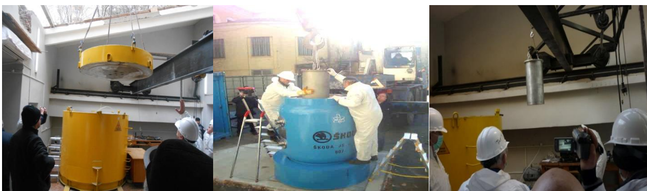
Fig. 12 Dismantling of the subcritical assembly
