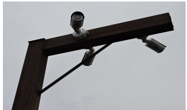
Fig.33 View of radiological and video monitoring system at Saakadze site
