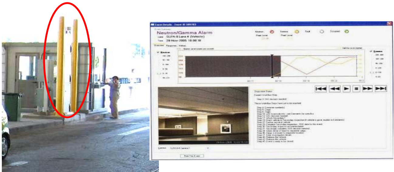
Fig. 34 View of portal monitor and report print out
