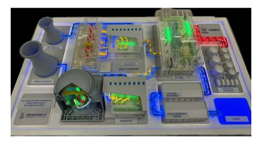
FIG. A.10. Model of the phase 1 Jiangsu Xuwei nuclear power heating plant project, with two HPR1000 reactors (one unit shown in foreground) and one HTR-PM600S (six reactors shown in the centre), as presented to the Agency. (Source: IAEA)
