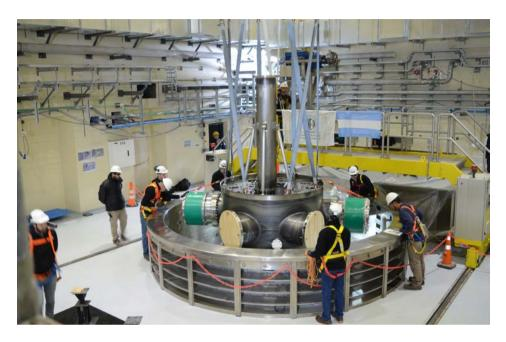
FIG. E.1. Installation of the reflector tank at the RA-10 research reactor, Ezeiza Atomic Centre, Argentina. (Source: National Atomic Energy Commission (CNEA), Argentina)
