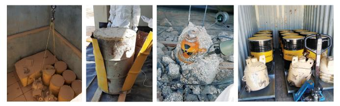
FIG. C-4. Retrieval and conditioning of radioactive sources in new waste packages at a legacy waste storage site in Jordan. (Photos: Jordan Atomic Energy Commission)
