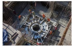
FIG. D-1 c. Installation of floor slab in the base of the MBIR reactor cavity, Research Institute of Atomic Reactors State Scientific Centre, Dimitrovgrad, Russian Federation. (Photo: Rosatom)
