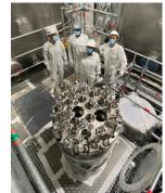
FIG. D-1 b. Installation of the closure head of the Jules Horowitz Reactor in Cadarache, France. (Photo: CEA).
