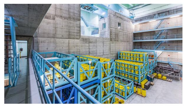
Storage hall for low- and medium-level radioactive waste at ZWILAG Switzerland. (Photo: ZWILAG Zwischenlager Würenlingen AG)
