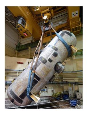
FIG. A-12. Removal of the last of 12 steam generators weighing 145 tonnes from the decommissioned Bohunice V-1 NPP in Slovakia. (Photo: Nuclear and Decommissioning Company JAVYS)
