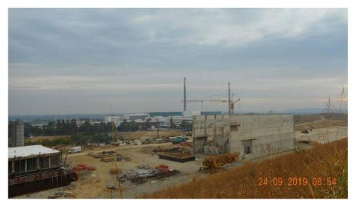
FIG A-17. Construction of the NDF at the Radiana site near Kozloduy NPP showing part of the administration complex (left), the waste reception and buffer storage building (right), and the loess-cement foundation of Disposal Platform 1 (far right).
