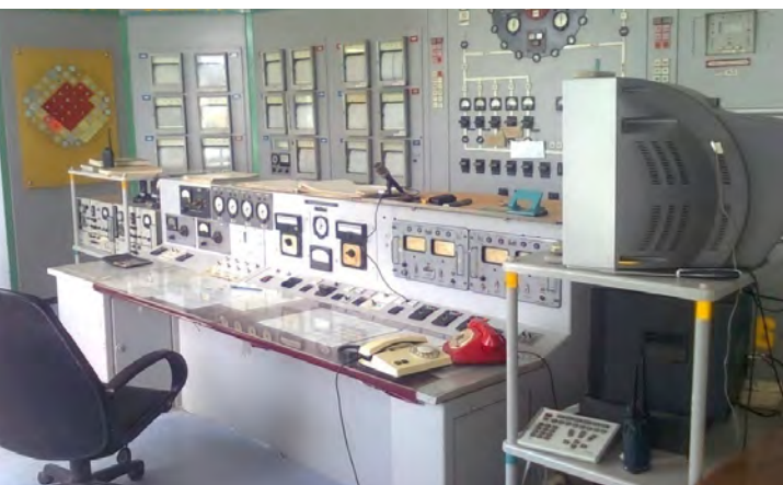
UZH9005: Instrumentation and control devices from the 1960s that were replaced with modern technologies.
