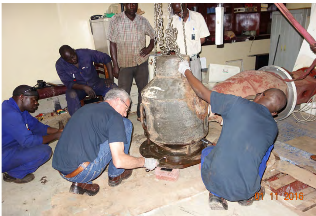
Decommissioning the old Cobalt-60 source at Mulago Hospital, November 2016.
