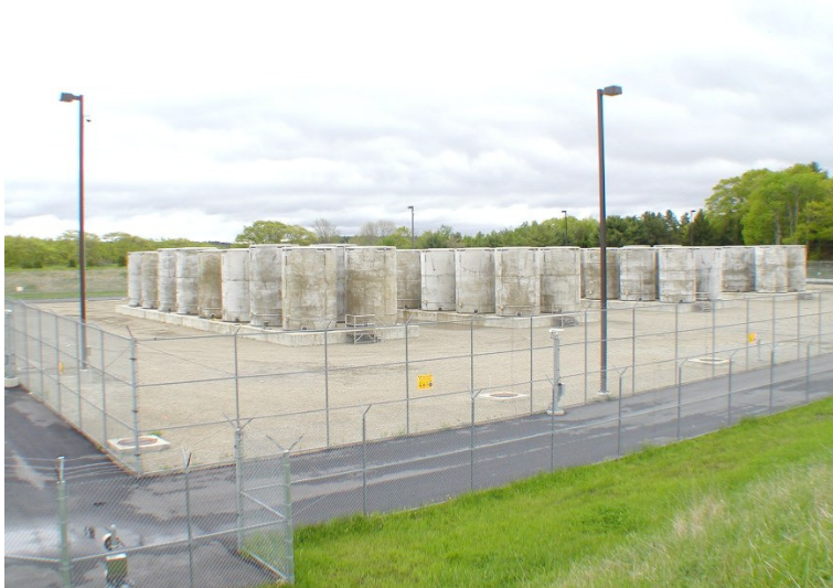
FIG. IV-4: The independent spent fuel storage installation at Maine Yankee
