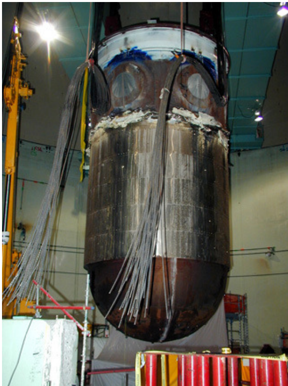
FIG. IV-2. Removal of the reactor vessel at Maine Yankee
