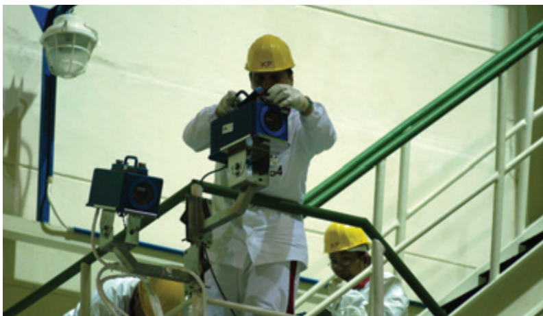
FIG. 2. Installing surveillance equipment at a nuclear facility.
