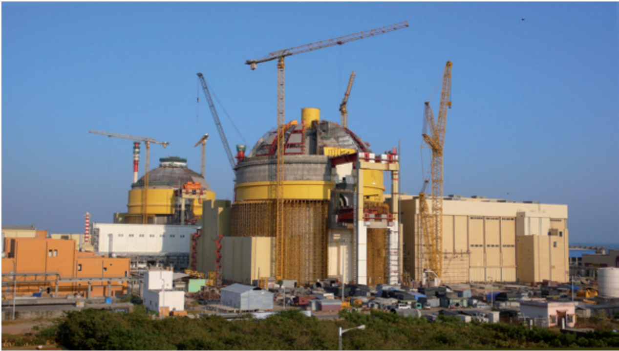
FIG. 1. Construction of water cooled reactors ( 2 \times 917 MW(e)) at Kundankulam, in India.
