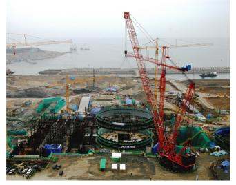
FIG. IV-9. Modularization of the containment liner plate assembly at Shin-Kori-1 in the Republic of Korea.
