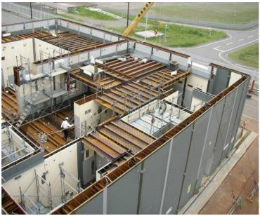
FIG. IV-11(b). Steel Plate Reinforced Concrete
