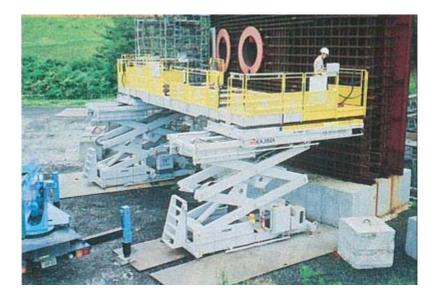
FIG. IV-12. An automatic scaffold and horizontal rebar feeding machine at Kashiwazaki Kariwa-6 in Japan.
