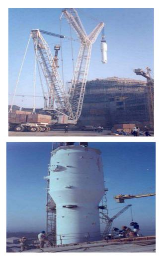
FIG. IV-5(a) and IV-5(b): Installing a steam generator at Tarapur-3, India.
