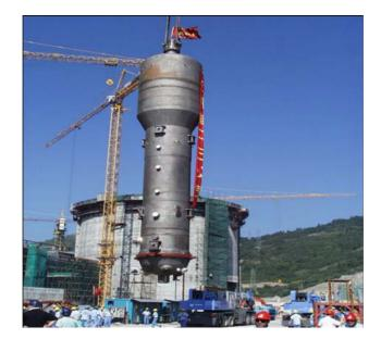
FIG. IV-2. Installing a steam generator at Qinshan 3-1 in China
